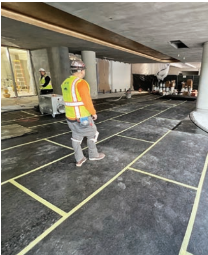
Rainbow Waterproofing's traffic coating
