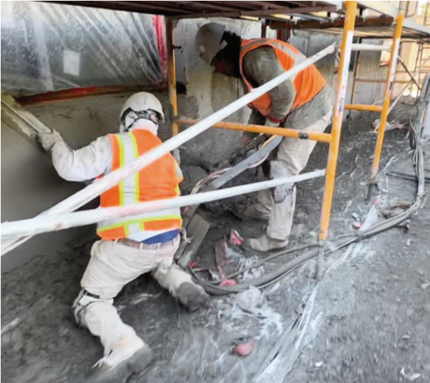
Local 300 plasterers work on the gun crew with Nevell Group at the Jefferson Adult Education Community Center in Daly City.
