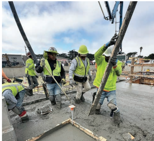
Local 300 cement masons work with R&R Maher Construction in Pacifica.
