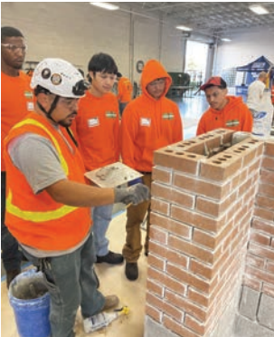
CTWI students repoint masonry.
